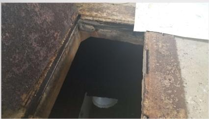
Hatch to climb under slow mix room – it is submerged in water and concrete is deteriorating
